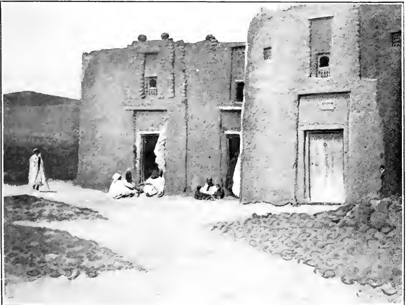
Laing's house, Timboctu.
